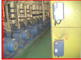
Install inverter at water pump
