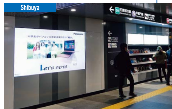
At the "Shibuya Station Big Signage," displays were installed without the use of protective cases. As a result, there are no glass cases in front of the screens and the high-resolution images are not lost.
