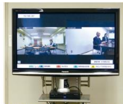
HDVC main unit, Camera, and display installed on a mobile Rack
