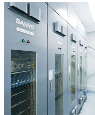
Power storage using a lithium mega battery system of the world's highest capacity class (1.5 MWh)
