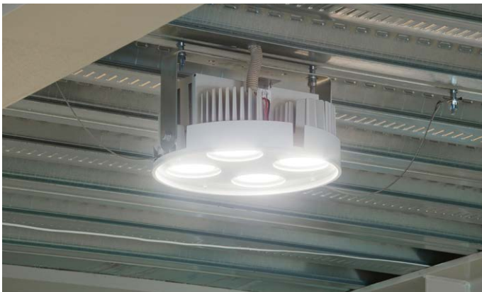
LED downlights in the factory building 2
