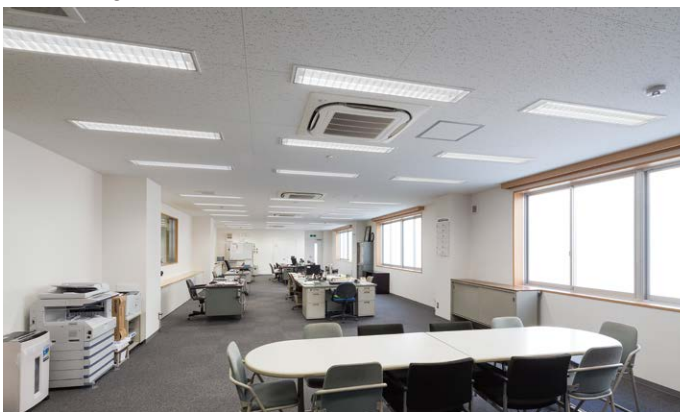
LED base lights in office areas
