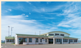
The Omagari Community Center with its base station antenna
