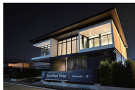
Modular building built on the premises of Thai Siam Steel headquarters in March 2021
