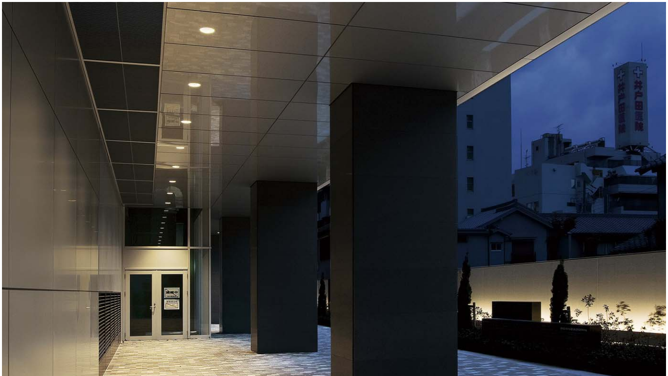
Nagoya Prime Central Tower
