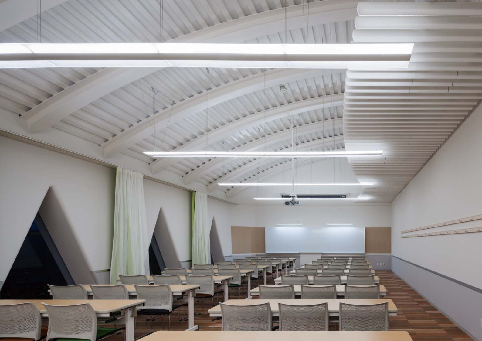
Sanko Gakuen Ayase School Building
