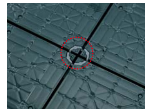
Earthquake-resistant connection rings prevent the panels from shifting.
